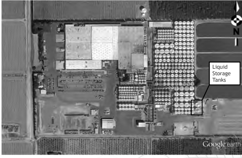
Wine Making Facility - Northern California
