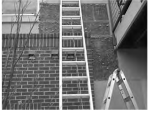
Exterior Veneer Removal
