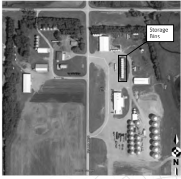
Storage Bin Failure Analysis - North Dakota (Google Earth 2014)
