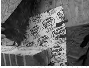
Exterior Veneer Removal
