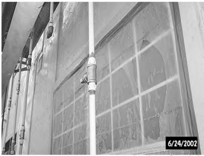
Water Spray Testing
