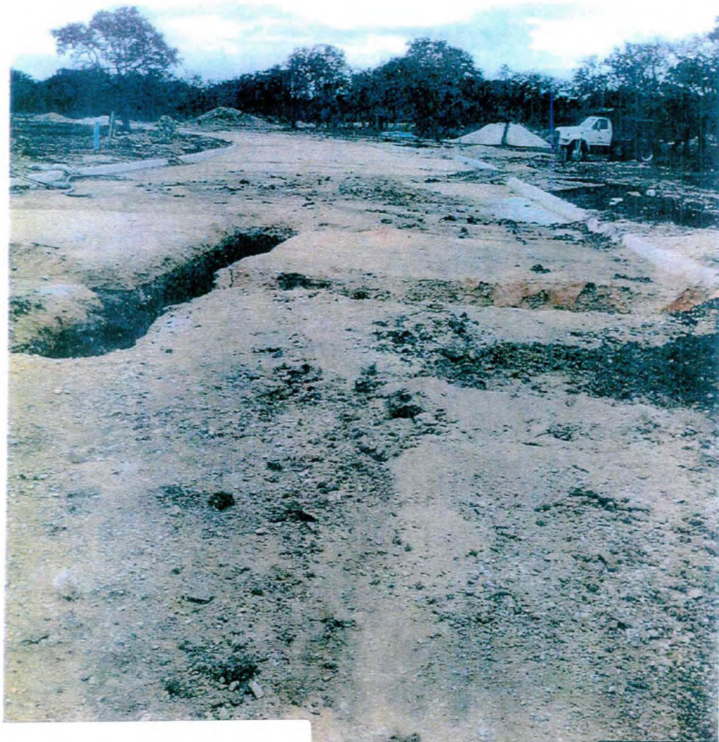
Trenching through road to access sewer main and sewer laterals.
