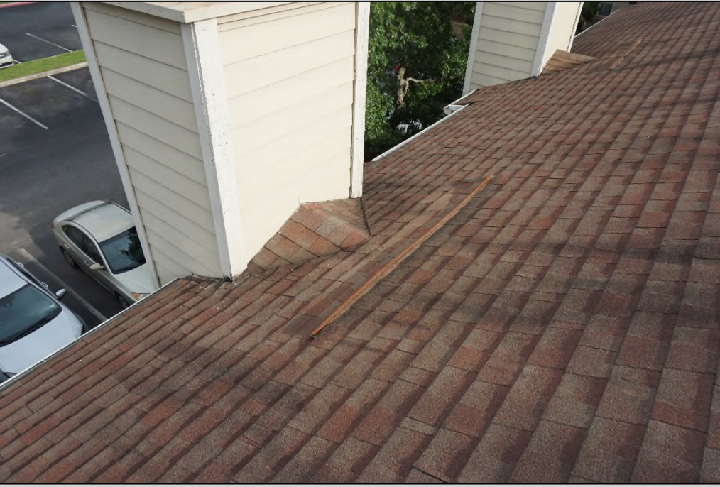
Figure 3-15: Wood cricket built on upslope of a chimney
