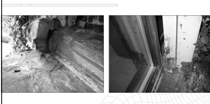
Openings Above Replaced Framing
