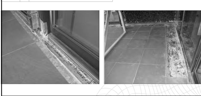
Removed Slate Pavers to View Wall and Terrace Interface
