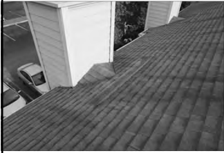
Figure 3-15: Wood cricket built on slope of a chimney
