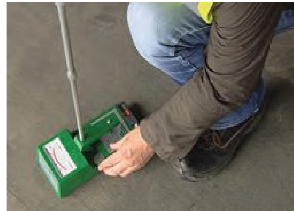
Electrical Capacitance (Impedance) Testing
