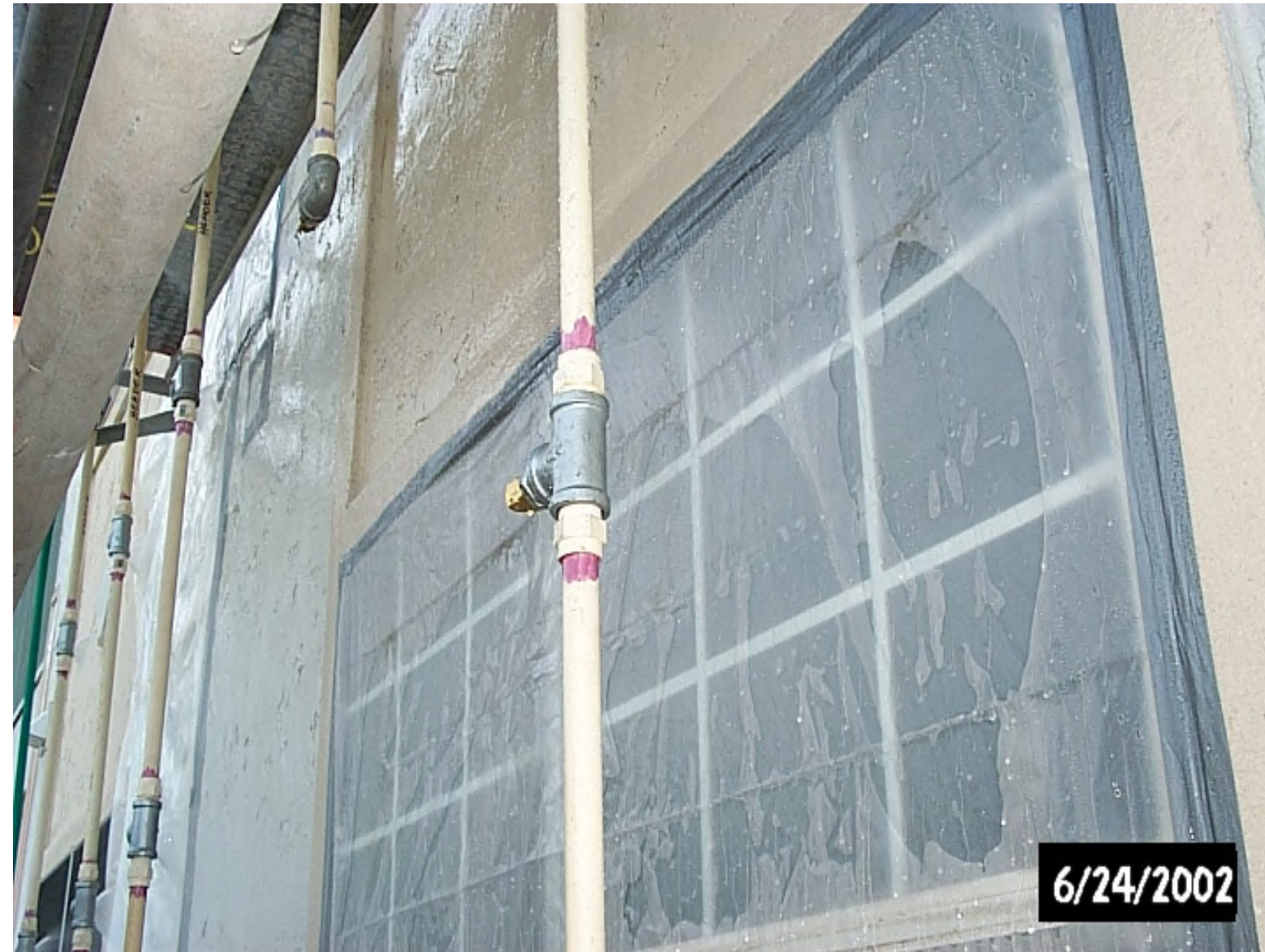
Water Spray Testing
