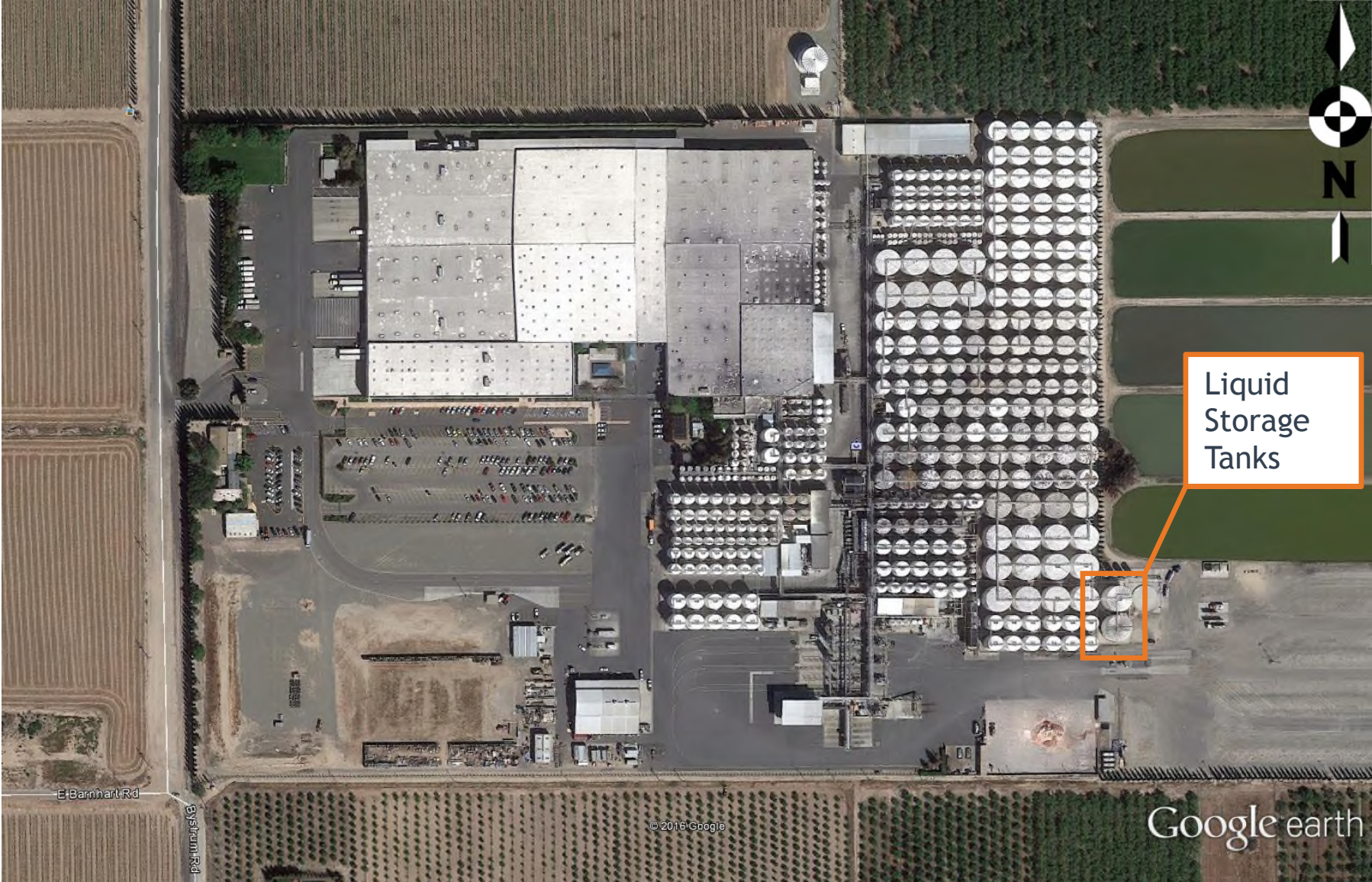
Making Facility – Northern California
