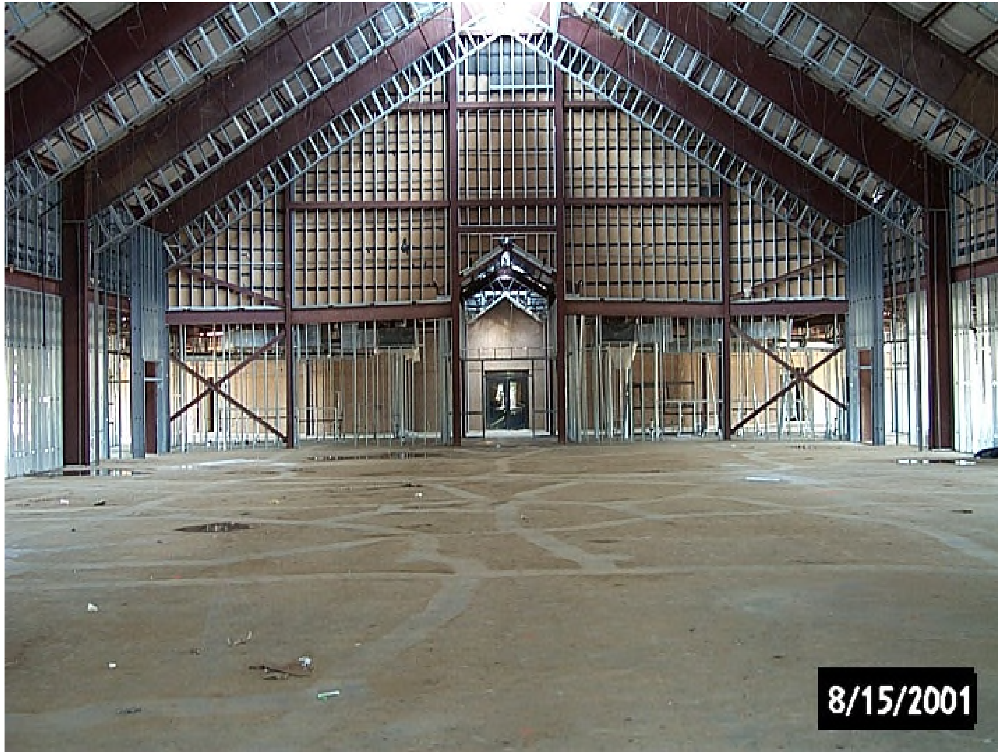
Broom Lines Remaining from Crack Mapping Survey
